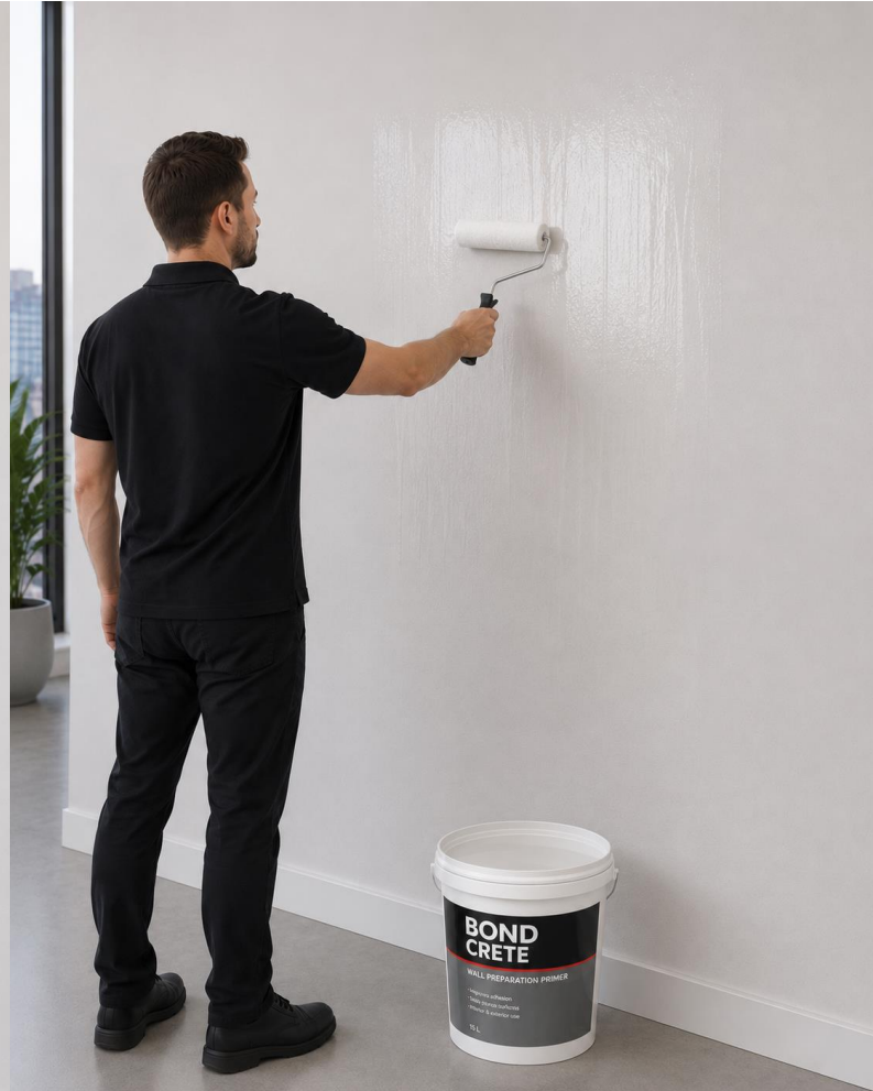
Step 2 Prime the wall with BondCrete or similar if required
