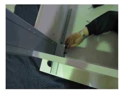
13. For additional support, add another screw through the hole in the plate on the transmission.
